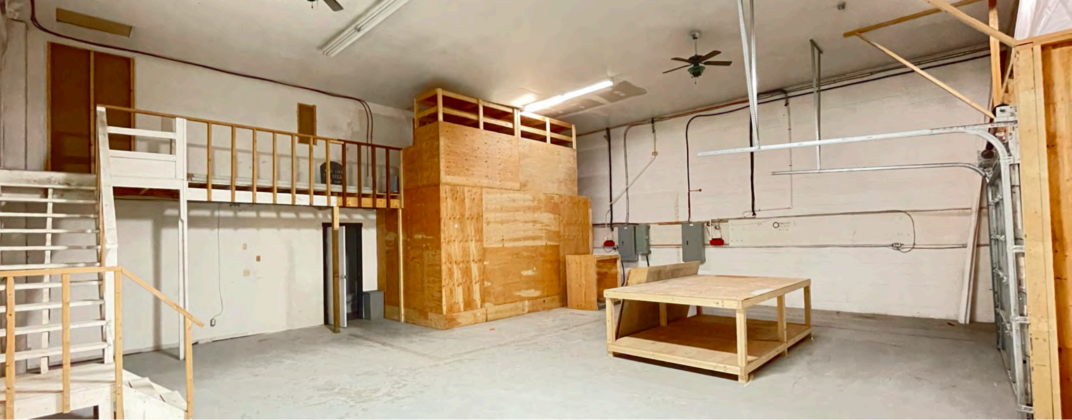
COMMON AREA LOADING DOORS FOR UNIT 5 AND 6
