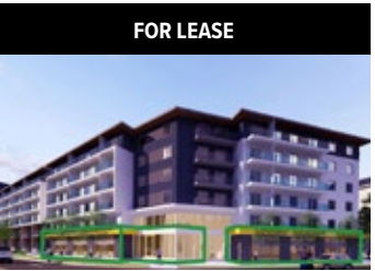
FOR LEASE CRU 1-3 2241 SPRINGFIELD RD, KELOWNA Victoria Mitchell, Jeff Brown Up to seven retail CRU's at Mission Heights, a 4.5 acre development which will house over 400 residential units.
