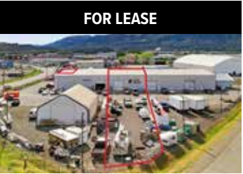
463 Dene Drive, Kamloops Marianne DeCotiis* ± 6,700 SQFT warehouse/office and yard space suited for trades, warehousing, and storage with indoor/outdoor functionality.
