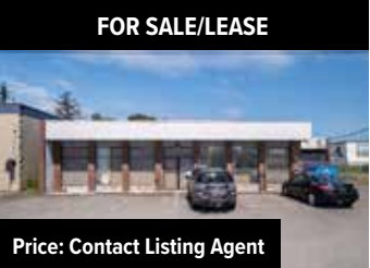
45951 Trethewey Avenue, Chilliwack Sam Repchuk ± 4,153 SQFT freestanding building with a warehouse and retail/showroom space, offering excellent exposure & accessibility.
